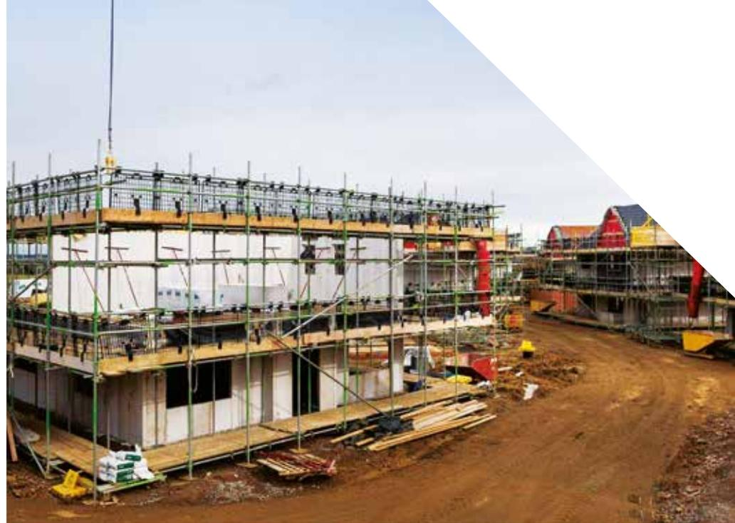
Celcon Elements are manufactured to the design storey height of the house with a width of 600mm and a thickness of 100mm. Elements are craned into place onto a bed of mortar on standard foundations. Vertical joints are filled with H+H element mortar – a fast-setting and very strong thin-layer mortar developed especially for use with the Elements and which forms a 2mm airtight joint.
