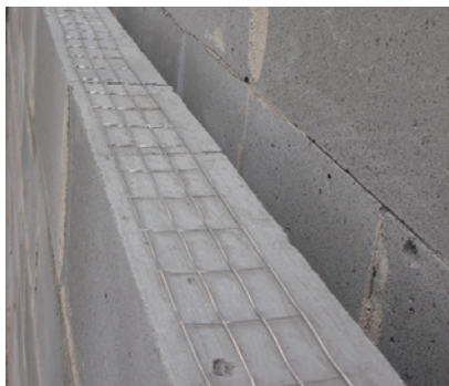
Bed-joint reinforcement
