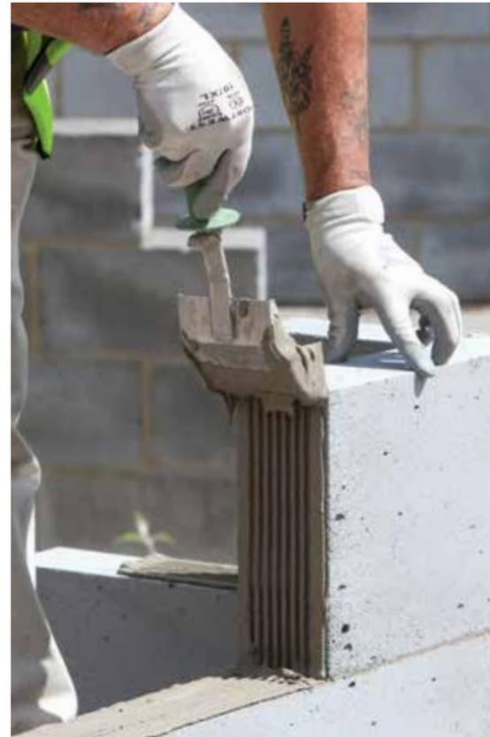
The Thin-Joint, Rå Build method of construction enables a fast, weathertight masonry shell to be built, allowing follow-on trades to start work sooner in a weatherproof environment, whilst retaining the flexibility of on-site construction. Thin-Joint is a recognised Modern Method of Construction and has been fully adopted as the preferred method of wall construction throughout most of northern Europe.
