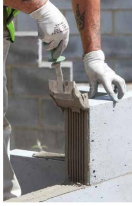
The Thin-Joint, Rå Build method of construction enables a fast, weathertight masonry shell to be built, allowing follow-on trades to start work sooner in a weatherproof environment, whilst retaining the flexibility of on-site construction. Thin-Joint is a recognised Modern Method of Construction and has been fully adopted as the preferred method of wall construction throughout most of northern Europe.
