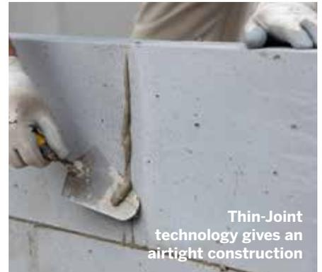
Thin-Joint technology gives an airtight construction
