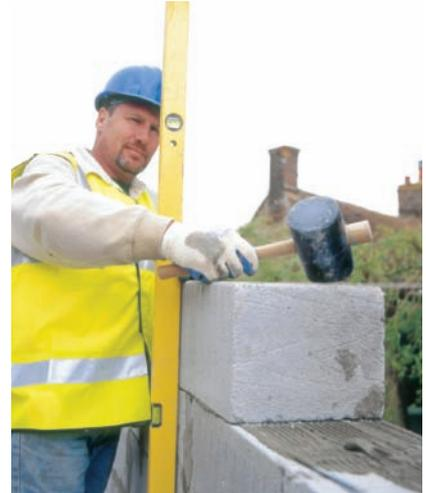
Thin-Joint technology gives an airtight construction
