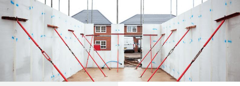
The H+H Vertical Wall Panels system is adaptable to suit most house designs and can be cut on site. If modifications have to be made once building commences, this system is completely adaptable, without going back to the drawing board or being subject to any extensive factory waiting times.
