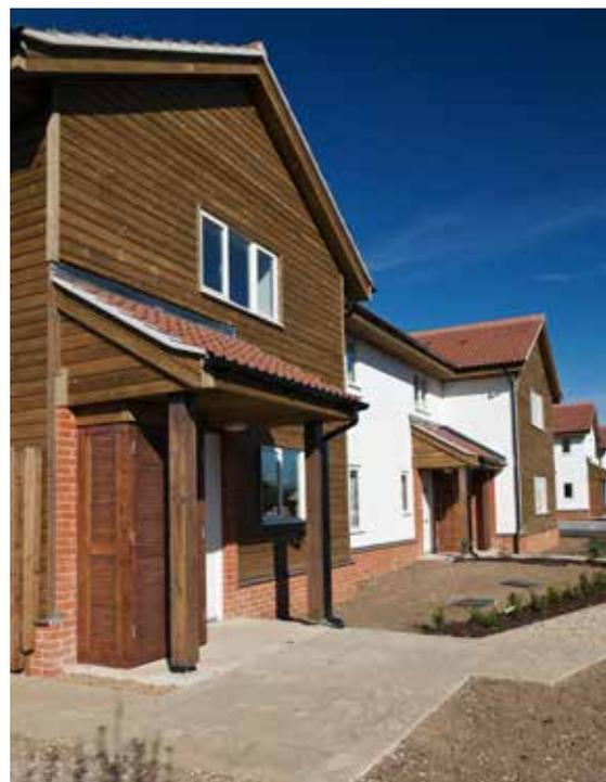
“We have been delighted to work on this project, our Rå Build method has proved popular within the Affordable Housing sector. Using a 140mm block as an alternative to timber frame shows how flexible aircrete can be. Solid wall provides a fast build speed, enabling a quicker weather-tight masonry shell to be built allowing internal trades to start sooner.”
