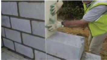
Straight, un-bonded vertical joints are the most common type of movement joint, and can be formed by butting the H+H aircrete blocks against both sides of a strip of rigid or flexible filler (such as polyethylene foam). A flexible sealant may be applied as required to maintain air tightness.
