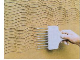
Newly applied rendering should be kept damp for the first day or two and the next coat should not be applied until the undercoat has adequately dried for a further two or three days. It is necessary for the drying to take place to provide suction for the next coat. For three-coat work, the second coat should be approximately 9mm.
