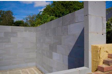
Aircrete is an excellent all round commercial and industrial building material. Used in partition and external walls (both solid and cavity), fire walls and as infill to steel and concrete framed buildings it provides durability, fire resistance and superb thermal and acoustic insulation.
